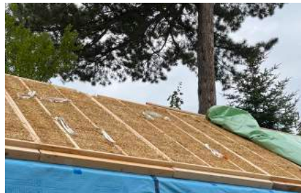
Gersdorf school building, 12 tons of CO 2 secured.
